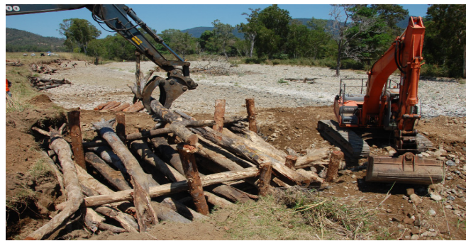
Constructing Engineered Log Jam No. 3
